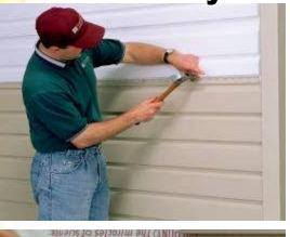
"Hang" the siding like you normally would. DO NOT NAIL TIGHT. You should be able to slide the vinyl siding panel horizontally after nailing.
