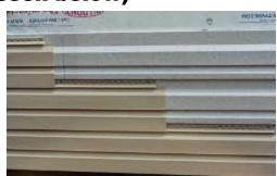
Nail the vinyl siding panels through the FULLBACK.
