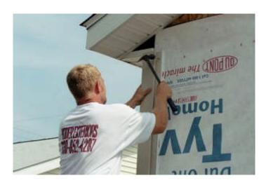
B. Insert Inside EasyPost corner behind the vinyl inside corner. Nail through vinyl nailing flange.
