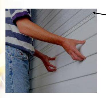
To insure the vinyl siding panel and the FULLBACK panel maintain their proper alignment, make sure the distance between the top of the vinyl panel's nailing hem and the FULLBACK panel's butt, above the hem, are of equal distance along the panel before nailing.
