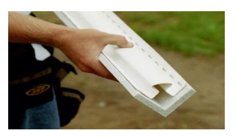
C. Cut the lineal to size and insert the FULLBACK support piece before locking into place and nailing.
