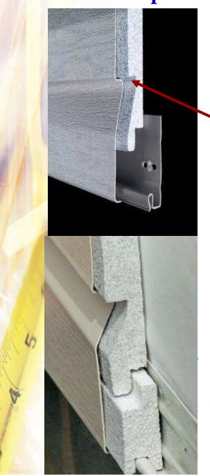
A. Attach the vinyl siding panel to the starter strip, then before nailing the siding, rotate the top of the panel away from the wall and drop a FULLBACK foam panel behind the siding.
